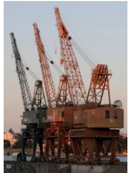
Cranes in the evening light poised to return to work at Drydock One, listed on the National Register of Historic Places at the former Mare Island Naval Shipyard.
